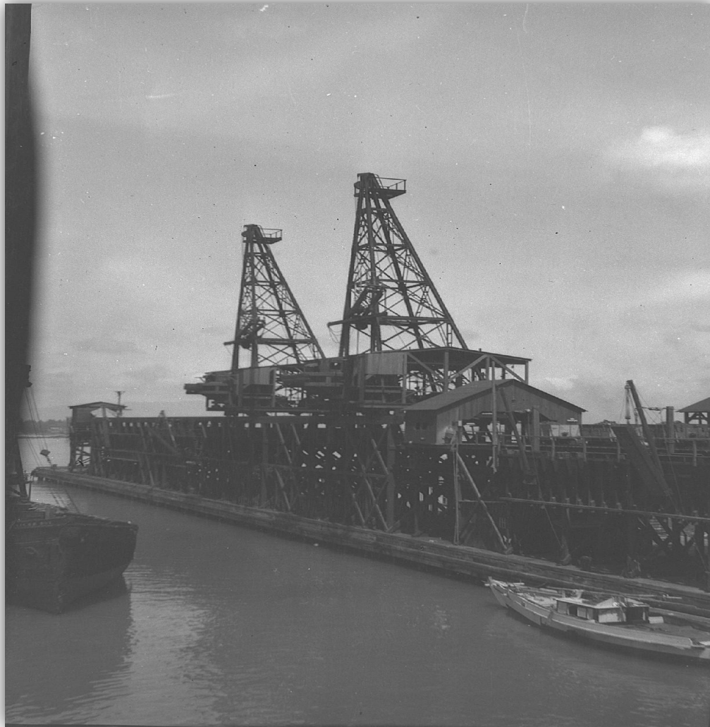
Dry Dock #1 under Construction nd.
