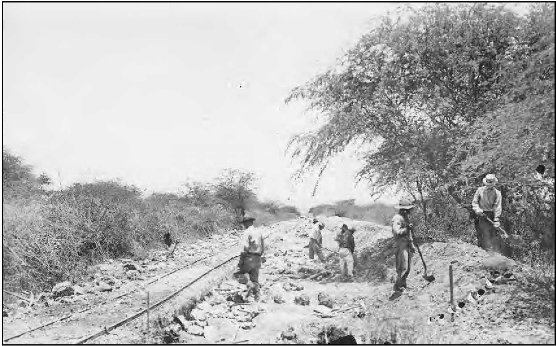
Construction of Temporary Railroad Spur to Watertown ca. 1909
